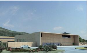
The Penitentiary Center Norte 1 is composed of a set of buildings which cover the different functions which have been projected and from a structural point of view consist of a group of independent buildings which form one unit interconnected via walls and galleries.
